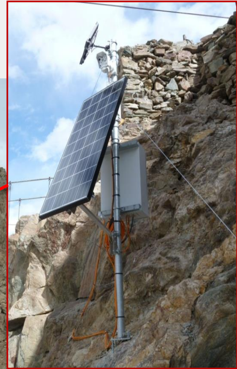
Control unit: data logger, 2 cameras, satellite communication unit, weather station, solar panel
